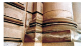
Efflorescence
