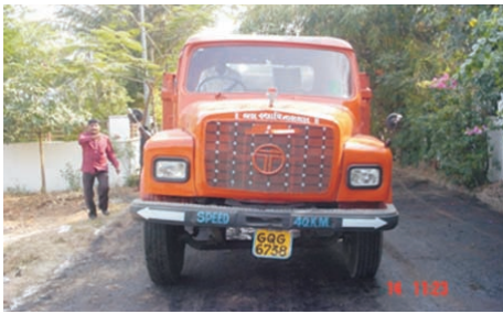
With Nanotac: No pick up just 15 minutes after application
