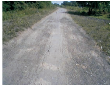
Control - Stripped asphalt surface with cracks and depression
