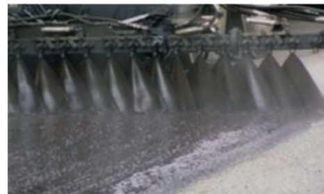
With Nanotac - Clean Nozzles, Uniform Spray
