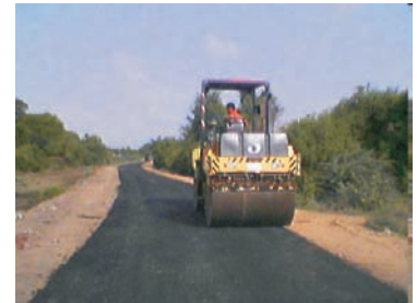
Compaction of Zycosoil modified asphalt layer
