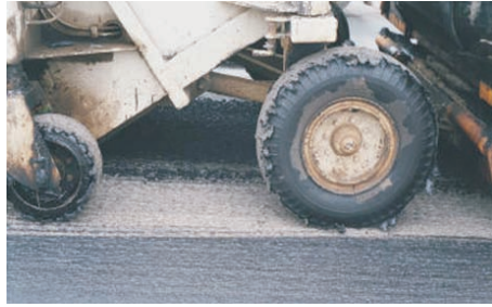
Without Nanotac: Tire Pick Up
