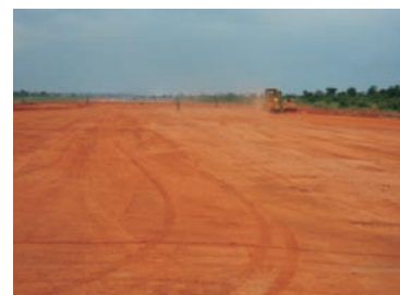
Untreated compacted soil layer
