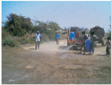
Spraying Terrasil solution on compacted bottom layer
