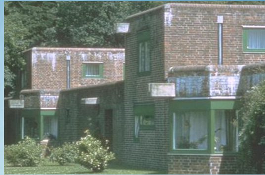
Efflorescence
